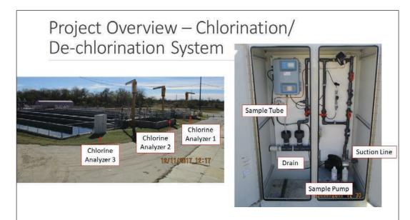
Automating the disinfection process at the Leon Creek Water Recycling Center reduced the facility's chemical use and saved operators many hours of manually monitoring and adjusting concentration levels.
