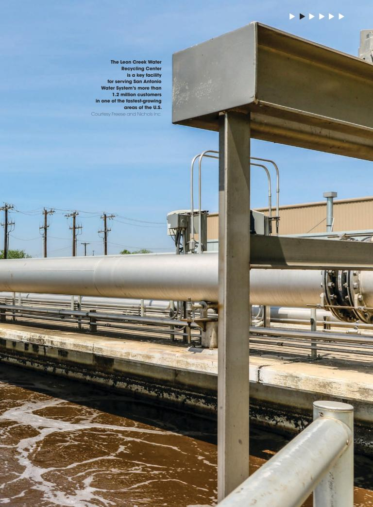
**Automating the** aeration system for the 15 basins at the Leon Creek Recycling Center corrected imbalanced air distribution, improved operations. and provided substantial cost savings for the San Antonio Water System. Courtesy Freese and Nichols Inc
